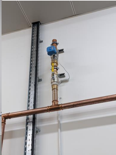
Over-pressure valve opens to atmosphere in event of compressor failure
