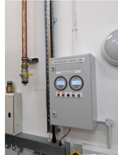
Over-pressure valve opens to atmosphere in event of compressor failure
